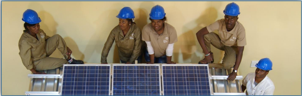
Training of UNAM & VTC Graduates at the Prosperita Facility (May, 2015) on a 23° Inclined Roof. Skills applied: Safety, Roof-tampering with the attachment of equipment and fixing of support/mounting structures to Trusses.
